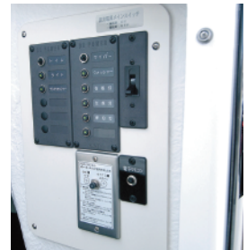
T. Breaker panel HK$1,400
